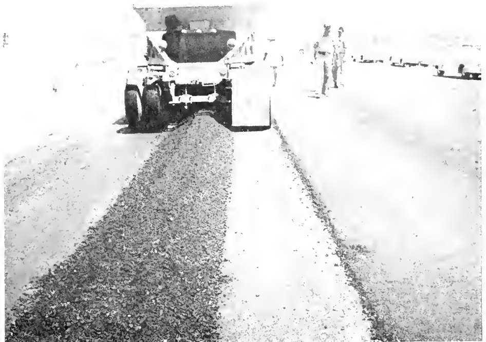
Windrow left by bottom dump hauling unit and special spreader box
